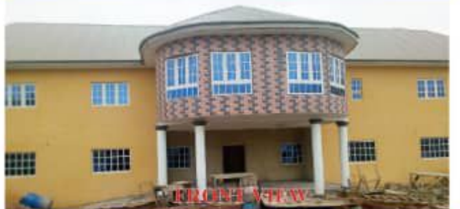
On-Going Office Complex (Front view) at NRCRI Umudike
