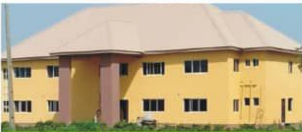
Professor Ukpabi Joseph Ukpabi Administrative Block At Igharim Sub Station
