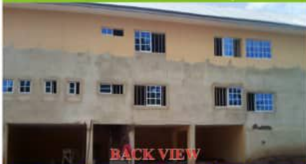
On-Going Office Complex (Back view) at NRCRI Umudike
