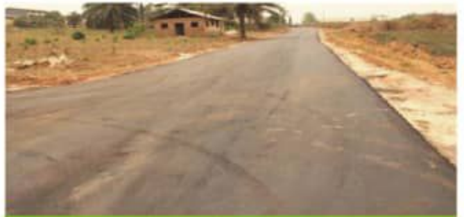
New Road Constructed at NRCRI Umudike
