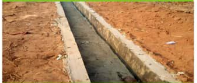
Water-way/Drainage System Constructed by E.D. in NRCRI, Umudike
