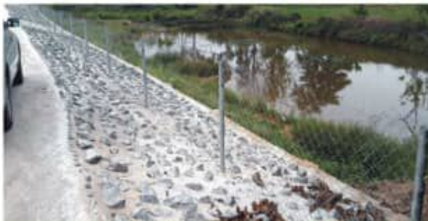
NRCRI Dam Erosion site restored by the E.D.
