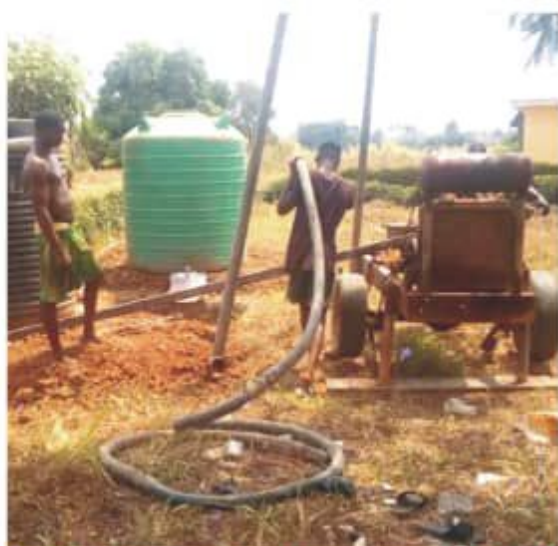
New Deep Water borehole executed by ED at NRCRI Igbariam
