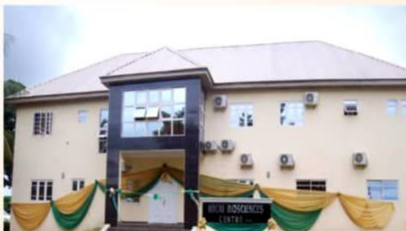
NRCRI New Biosciences Centre Building
